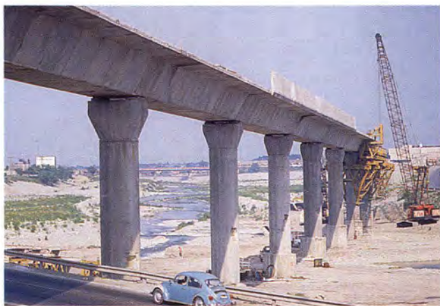
Fig. 9. The Metro line crossing of the normally dry Santa Catarina River is on high-level, skewed columns.
