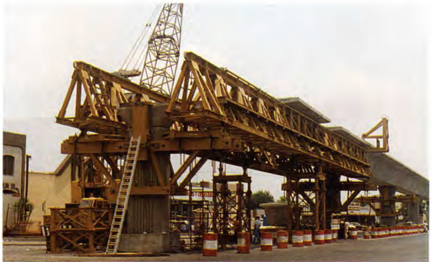
Fig. 19. Full-span erection trusses support the segments for a span until all are placed, post-tensioned and set on the pier bearings.
