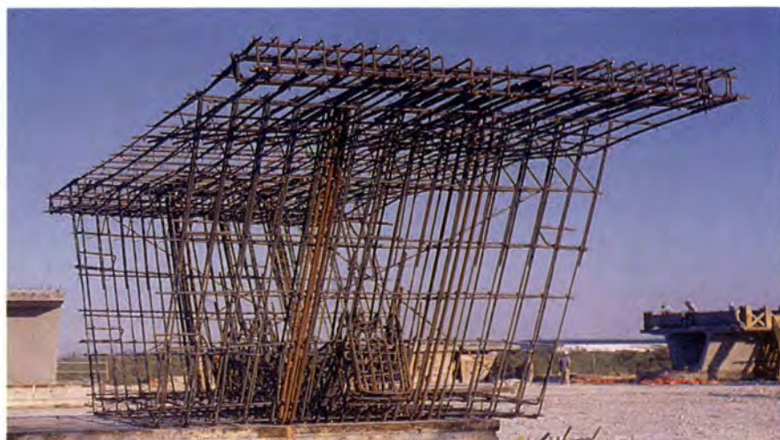
Fig. 12. Reinforcing bar cage for a typical segment.
