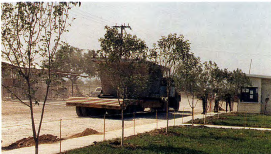
Fig. 18. A completed segment is hauled on a low-boy trailer from plant to bridge site.
