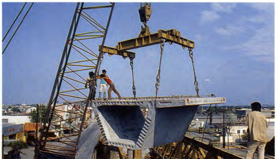
Fig. 21. Segments are lifted from street level by crawler cranes and set on erection trusses.
