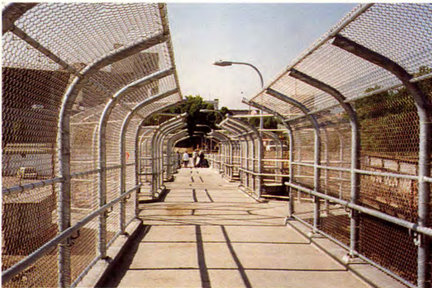
Fig. 15. Pedestrians' perspective of overpass.
