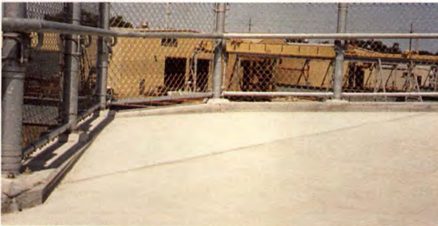
Fig. 8. Half-hexagon, cantilevered level landing.
