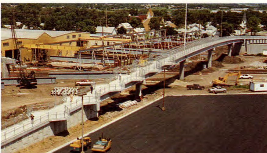
Fig. 16. Completed pedestrian/bicycle overpass looking northwest.
