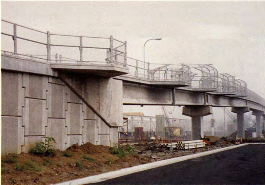
Fig. 2a. Mechanically stabilized earth (MSE) wall aesthetics.
