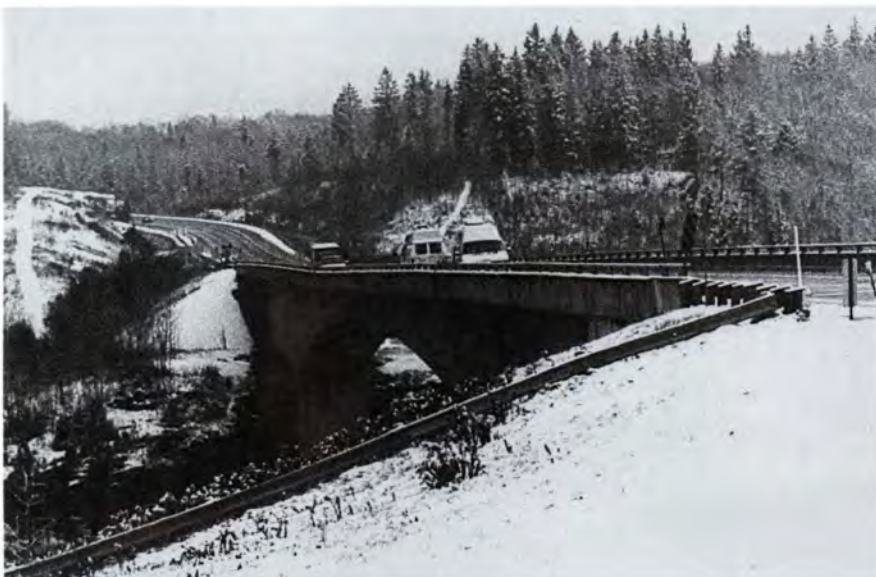
Fig. 6. Mobile bridge testing vehicle.
