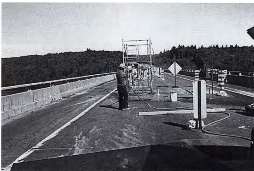
Fig. 21. Bridge strengthening operations, working from deck.
