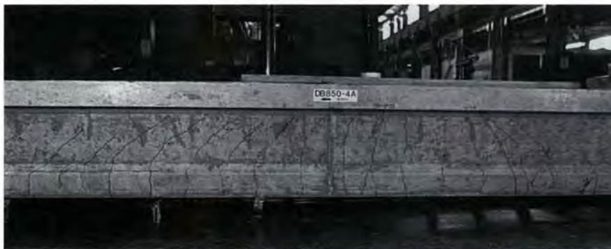
Fig. 16. Cracking pattern for Test DB850-4A — Typical for flexural failures.
