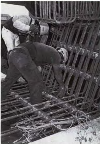
Fig. 6. Installation of thermocouples in segment prior to casting.
