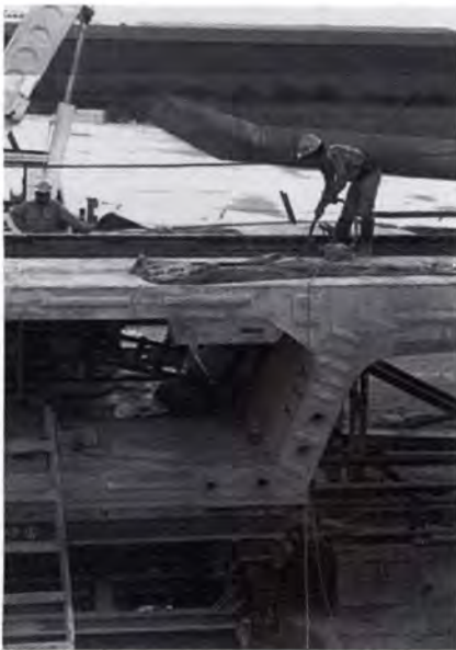
Fig. 1. Match casting operations.
