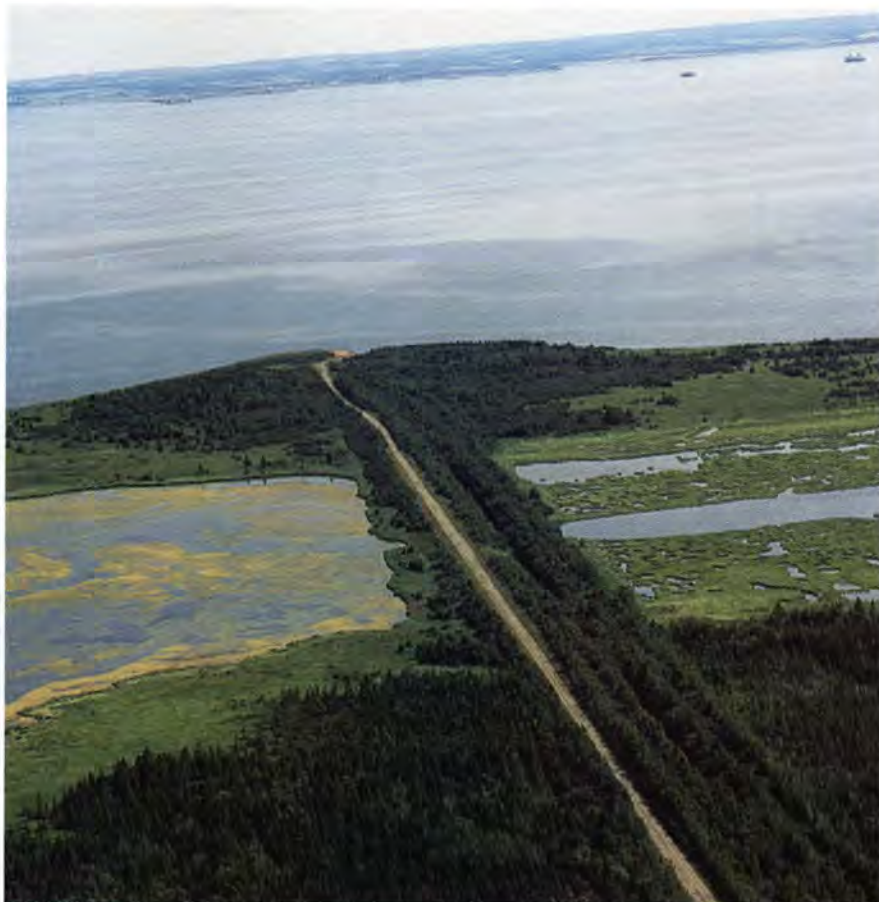
Fig. 4. Prince Edward Island in background; New Brunswick approach constructed in 1967 in foreground.
