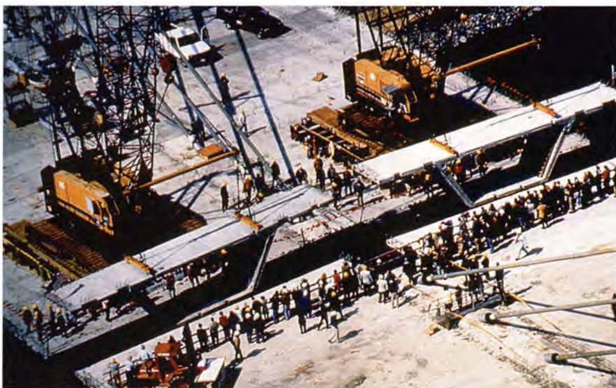
Fig. 17. Placement of final two box girder segments.
