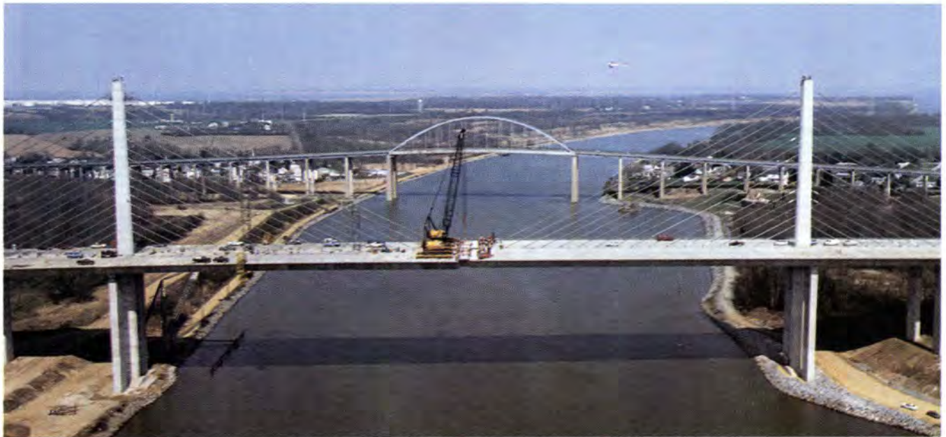
Fig. 1. Chesapeake & Delaware Canal Bridge. The last two segments were placed in the 750 ft (229 m) cable-stayed main span on April 3, 1995.
