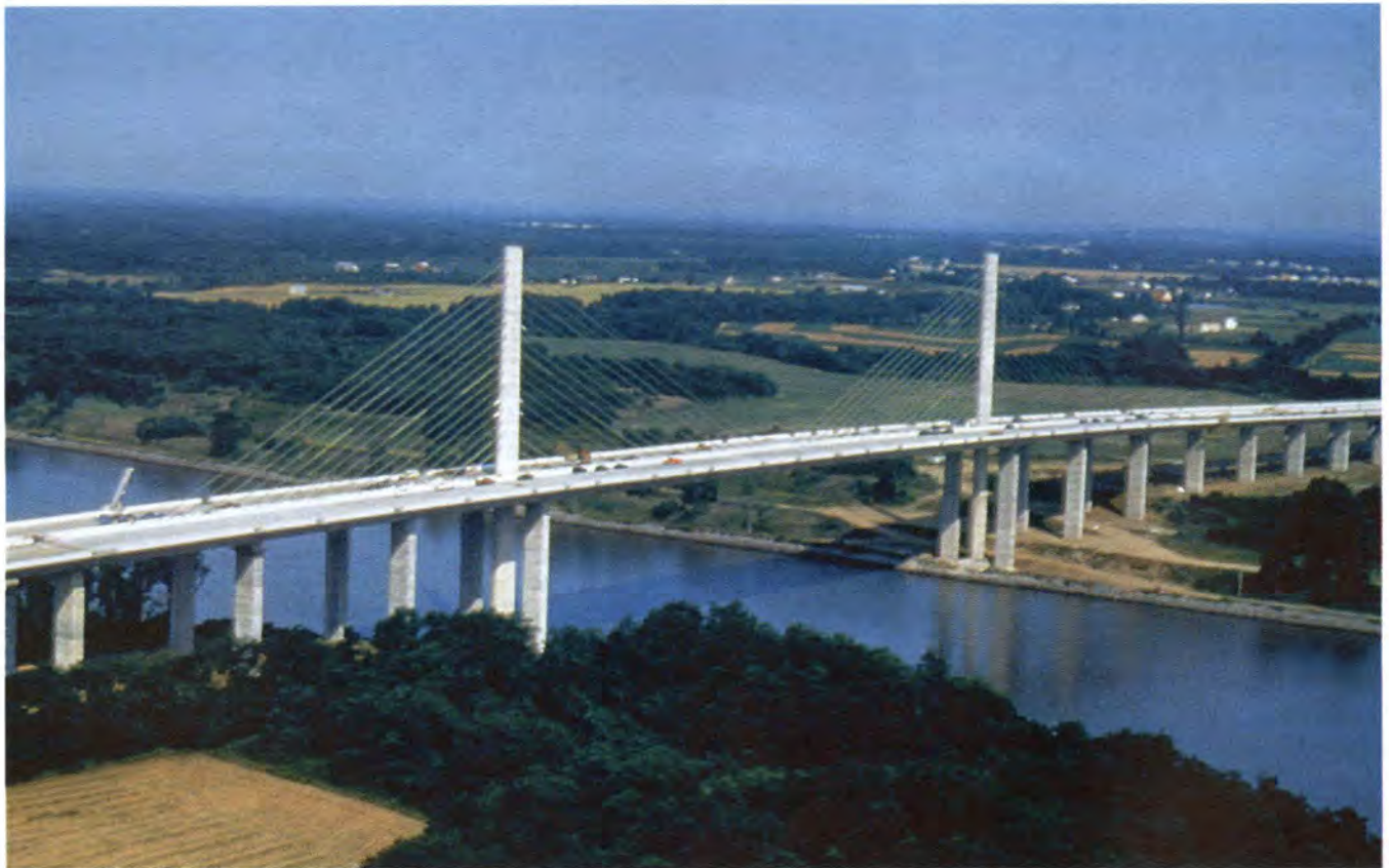
Fig. 18. Panoramic view of the nearly complete C&D Canal Bridge.
