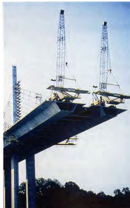
Fig. 14. Twin 200-ton (181 t) crawler cranes positioning trapezoidal box girder segments.
