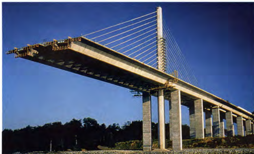
Fig. 15. Precast box girder segments cantilever from one of two main pylons.
