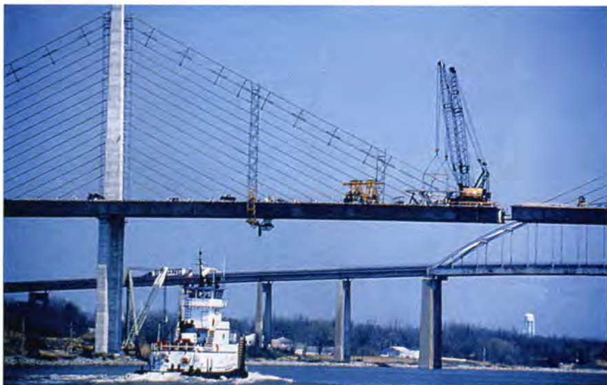
Fig. 16. Marine traffic proceeds unimpeded while construction continues above.
