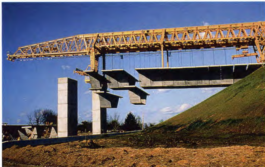
Fig. 13. Approach span erection truss moving several precast box girder segments.
