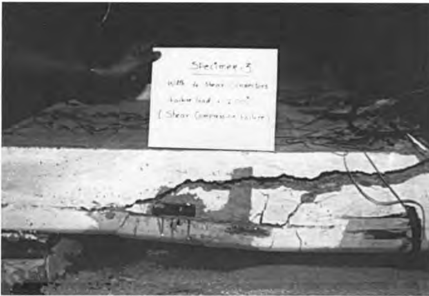
Fig. 17. Failure mode of Specimen 3.
