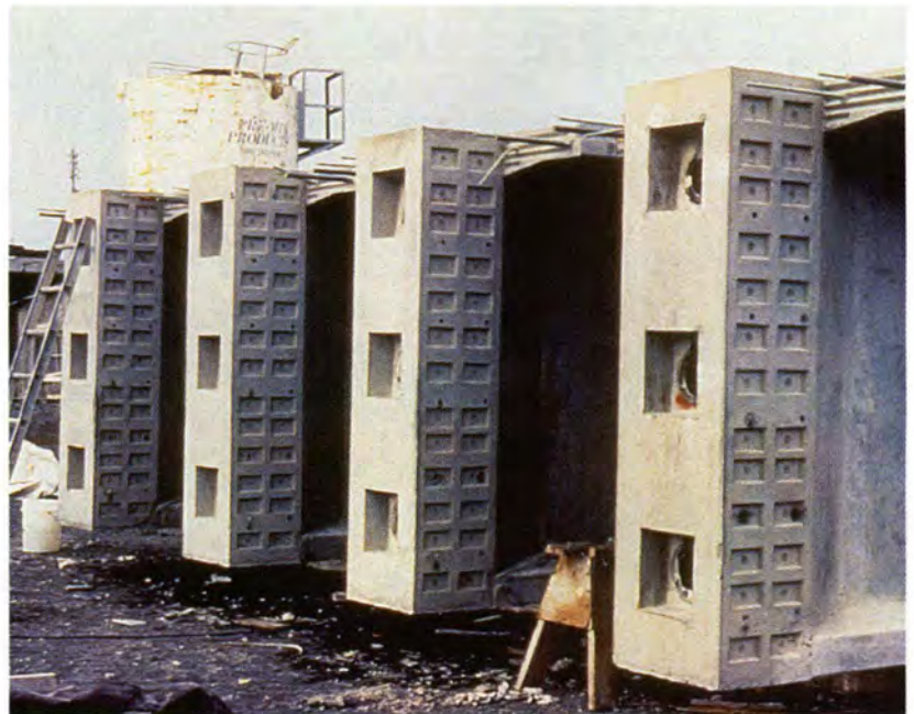
Fig. 10. Four girder end segments ready for shipment.
