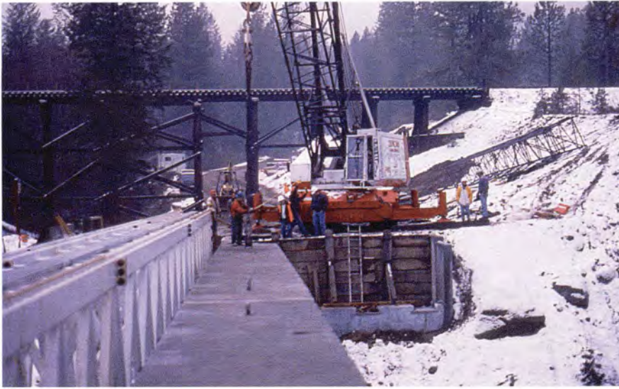
Fig. 22. Girder clear of launching truss being set in place.
