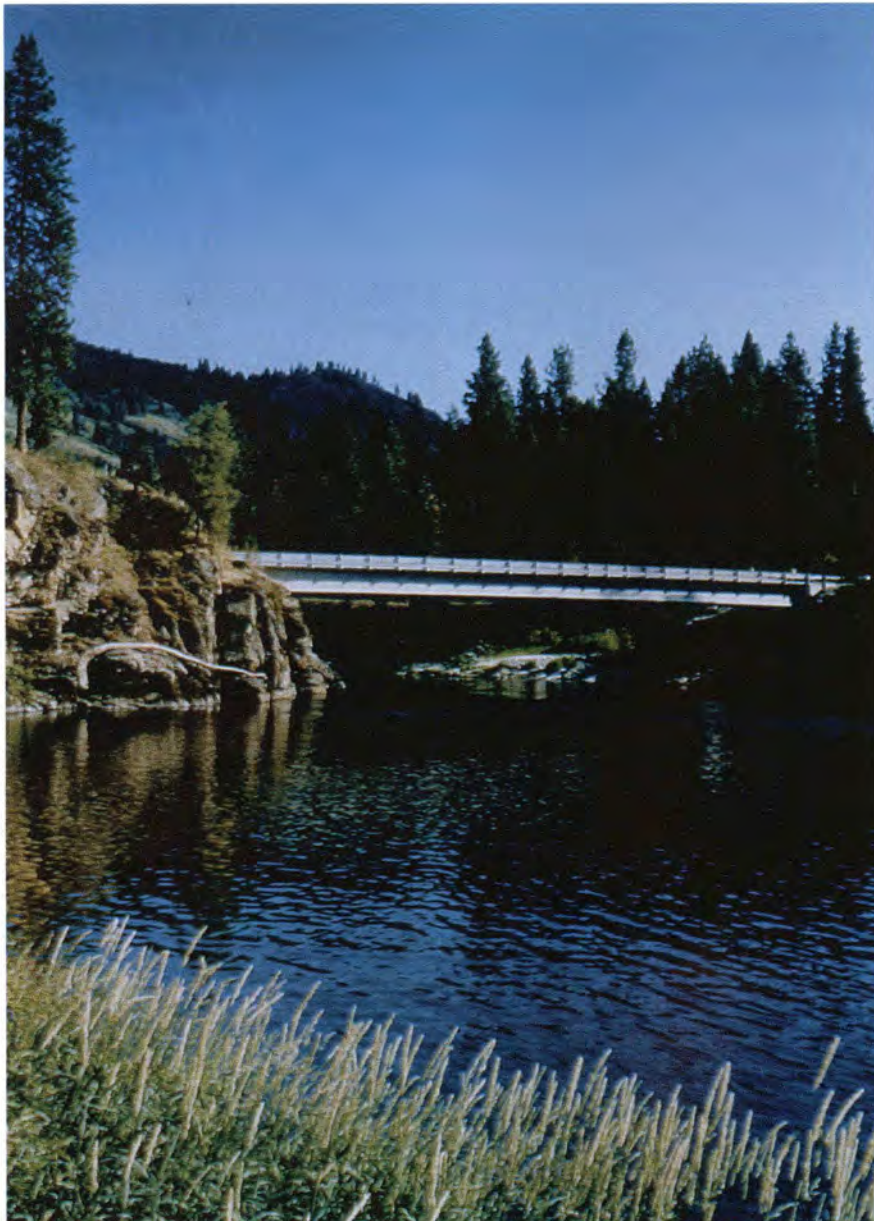
Fig. 23. Finished bridge as seen this past summer.
