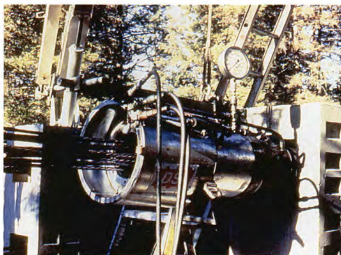
Fig. 14. Jacking the 190 ft 6 in. (58.1 m) girders after curing of closure pour.
