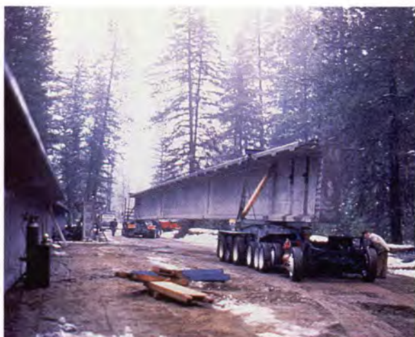
Fig. 17. Spliced girder [190 ft 6 in. (58.1 m) long and weighing 120 tons (110 t)] on the road and ready for the haul.
