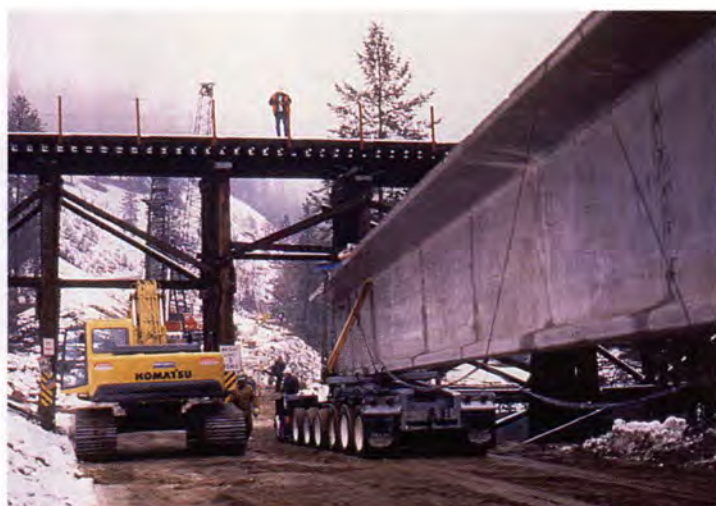
Fig. 18. Girder heading for bent opening specially modified for these girders.
