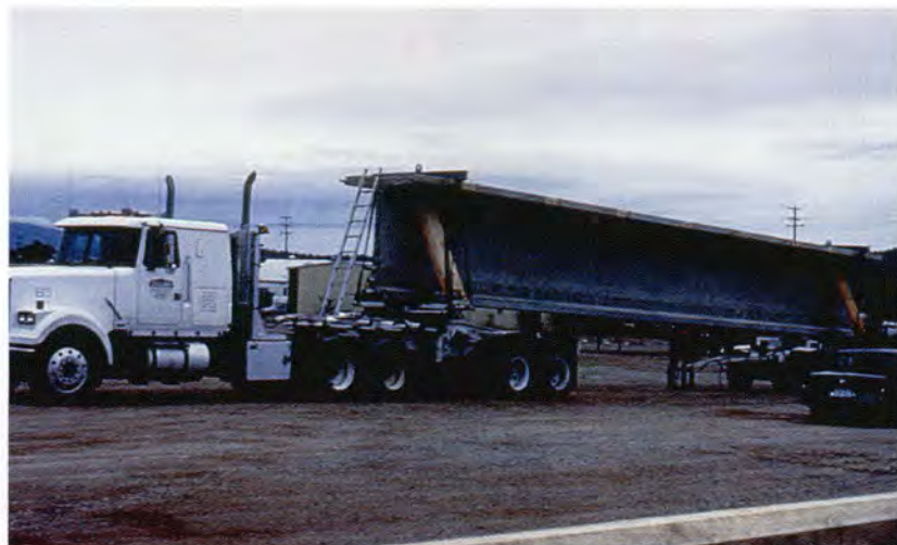
Fig. 11. Girder segment [63 ft (19.2 m) long and weighing 40 tons (36 t)] leaving precasting plant.
