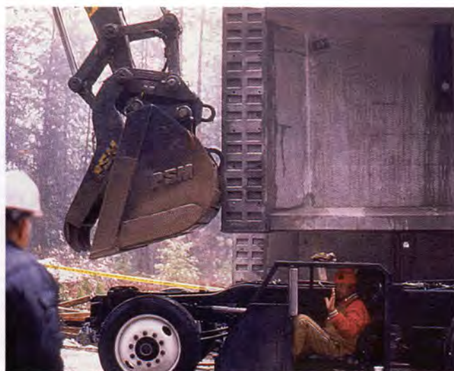
Fig. 16. Positioning spliced girder on seven-axle, 26-tire carrier.
