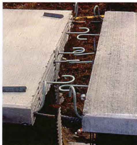
Fig. 12. Girder segments aligned at staging area near construction site.
