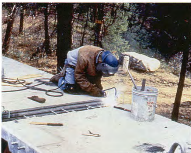
Fig. 13. Welding the outside #8 reinforcing bars at the closure segment.
