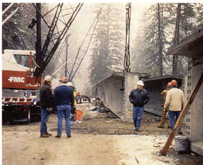
Fig. 15. Picking spliced girder in staging yard.
