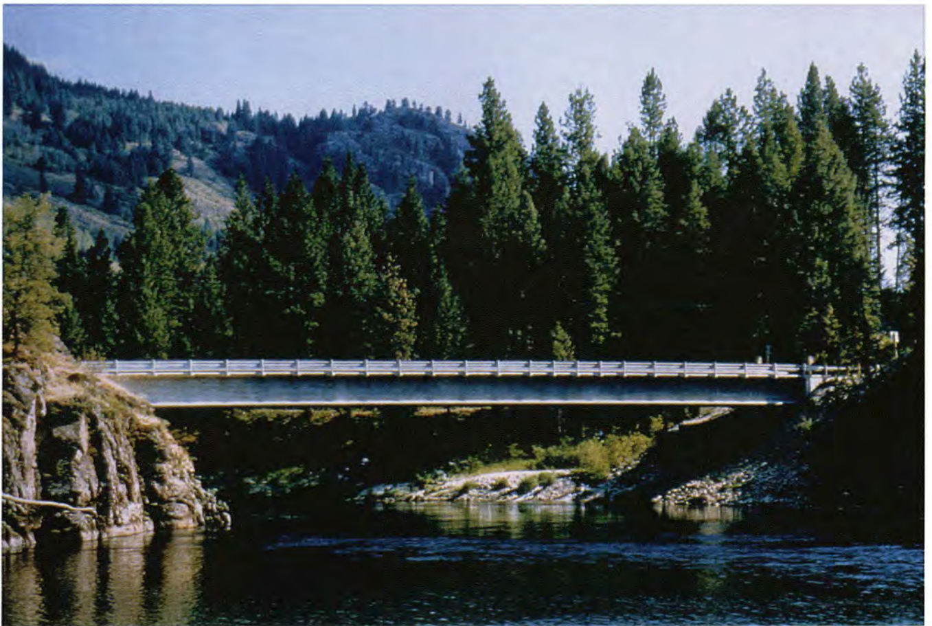
Fig. 1. Panoramic view of new Rock Cut Bridge.
