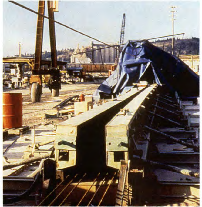
Fig. 8. Curing one 63 ft (19.2 m) girder segment after concrete was cast.
