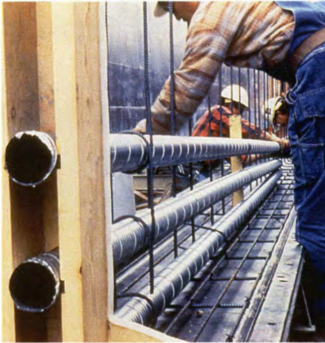
Fig. 7. Positioning post-tensioning ducts in one of the 63 ft (19.2 m) girder segments.
