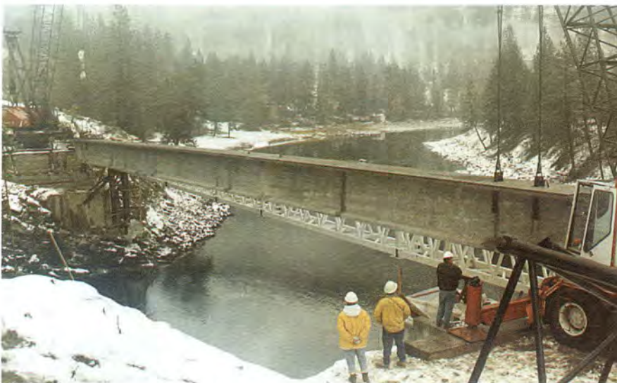
Fig. 21. Girder gently lowered into position on abutments.
