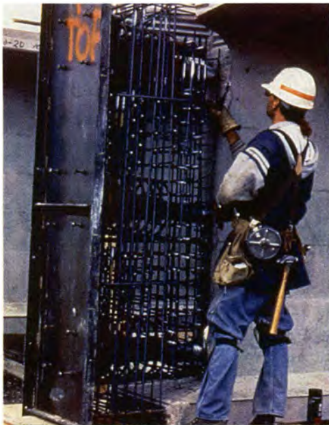
Fig. 9. Constructing girder and jacking cage after girder casting and curing.
