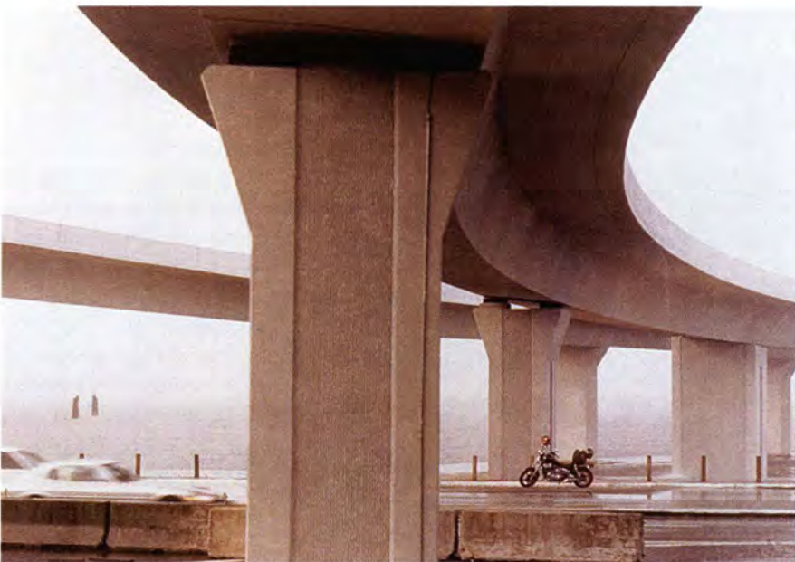
Fig. 12. I-110/U.S. 90 Bridge, Biloxi, Mississippi (Designer: Figg Engineering Group).
