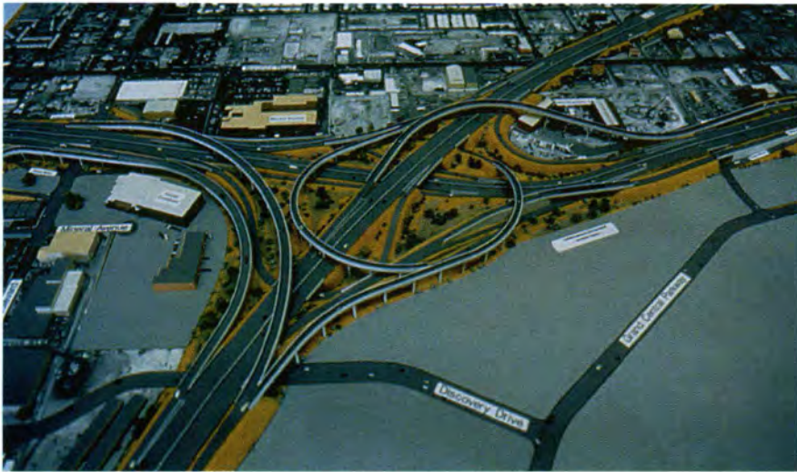
Fig. 18. I-15/U.S. 95 Interchange, Las Vegas, Nevada (Designer: Parsons Brinckerhoff).
