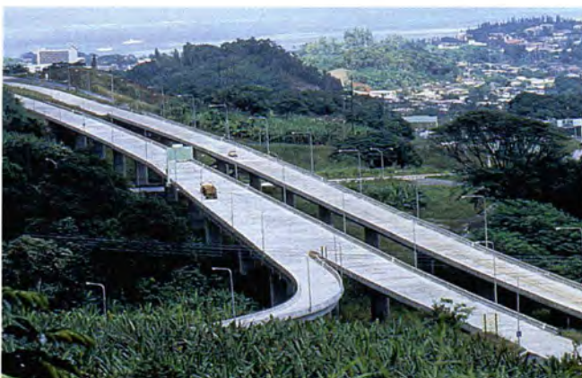
Fig. 13. Kaneohe Interchange Bridge, Oahu, Hawaii (Designer: J. Muller International).
