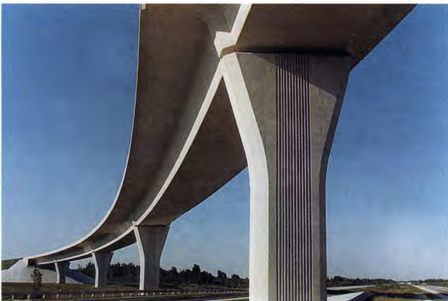
Fig. 10. Ramp 1, Florida — A precast segmental, post-tensioned, balanced cantilever viaduct (Designer: Beiswenger Hoch & Associates).
