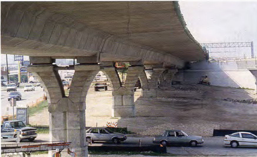
Fig. 15. U.S. 183 Viaduct, Austin, Texas (Designer: Texas Department of Transportation).
