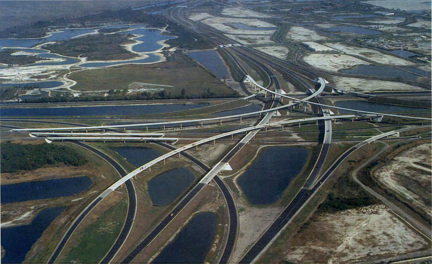
Fig. 1. I-75/I-595 Interchange, Broward County, Florida. This four-level fully directional interchange is the largest interchange in the state of Florida. The bridge structures are composed of curved precast concrete segmental box girders erected by the balanced cantilever method (Designer: Beiswenger Hoch & Associates).
