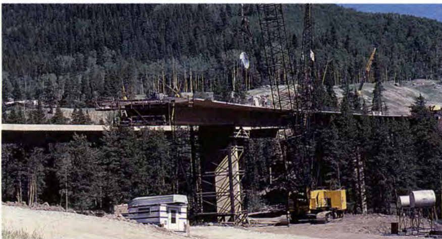
Fig. 9. Precast segmental construction at Vail Pass, Colorado, 1976.
