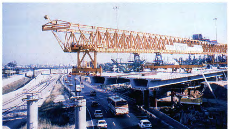
Fig. 7. Ayalon Interchange construction, Israel, 1995.
