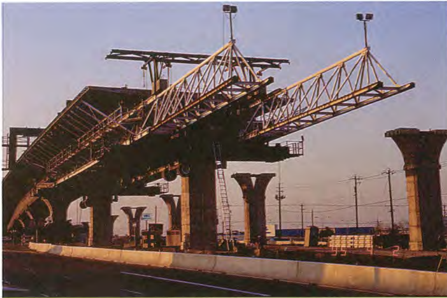
Fig. 4. Span-by-span erection, U.S. 183 Viaduct, Austin, Texas (Designer: Texas Department of Transportation).
