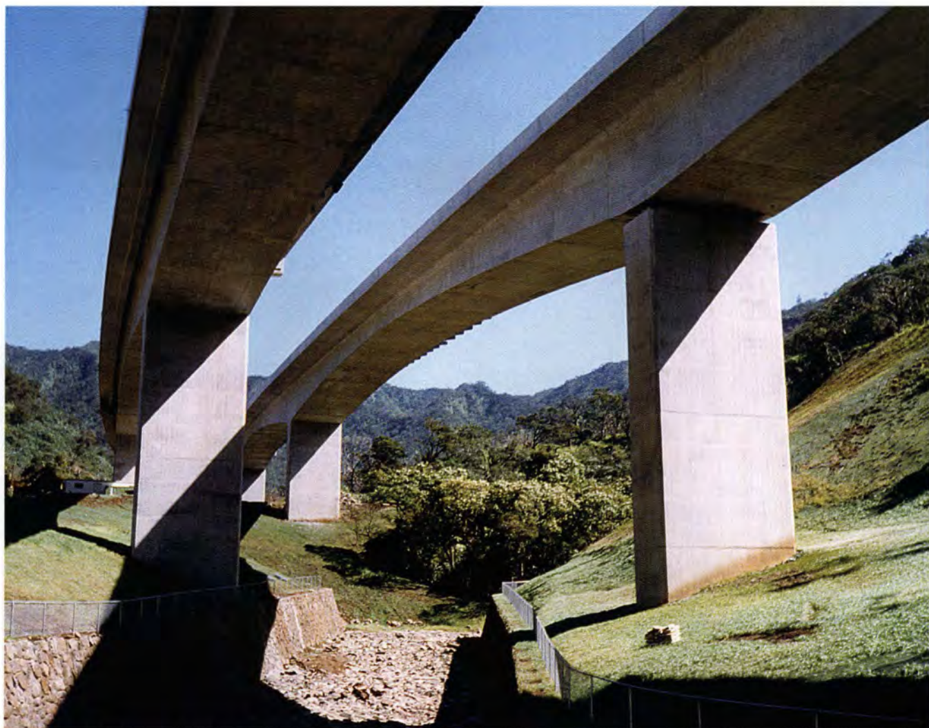
Fig. 1. North Halawa Valley Viaduct.
