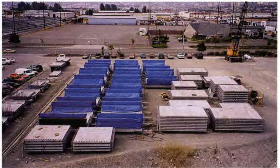
Fig. 11. Precast wall panels stockpiled and ready for erection.
