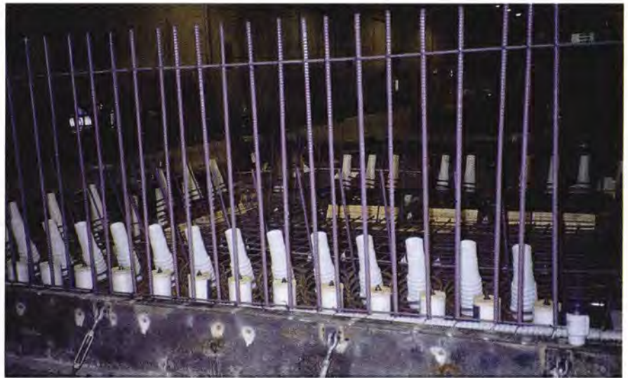
Fig. 10. Pontoon end wall form ready for concrete.
