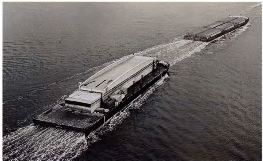
Fig. 27. Pontoon under tow to Hawaii behind a bargeload of prestressed girders. Note 250 ft (76.2 m) transition span riding “piggy back” on pontoon. (Courtesy: Crowley Marine Services. Photo by Lou VanDemark.)
