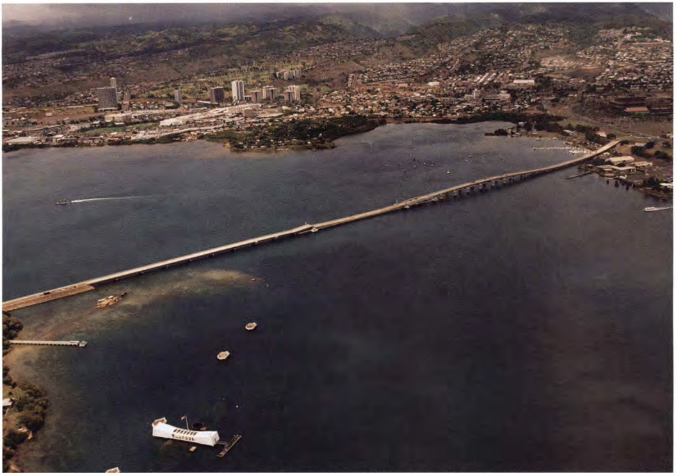
Fig. 32. Aerial view of completed bridge showing USS Arizona Memorial in left foreground. (Courtesy: Williams Photography of Honolulu.)
