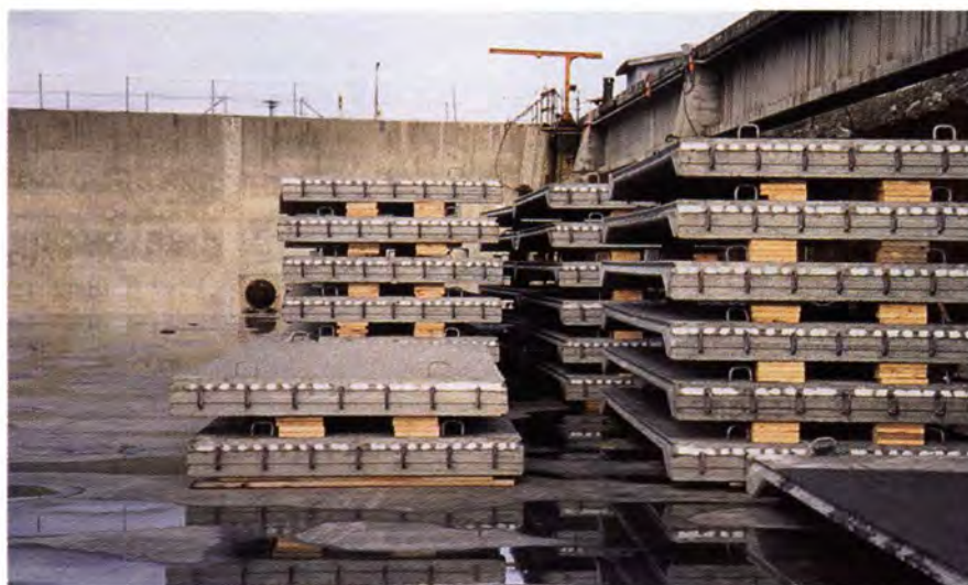
Fig. 15. Stockpiled haunched deck panels.
