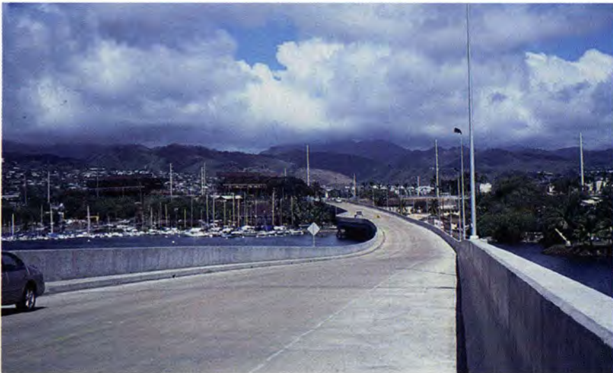
Fig. 29. Completed bridge looking east.
