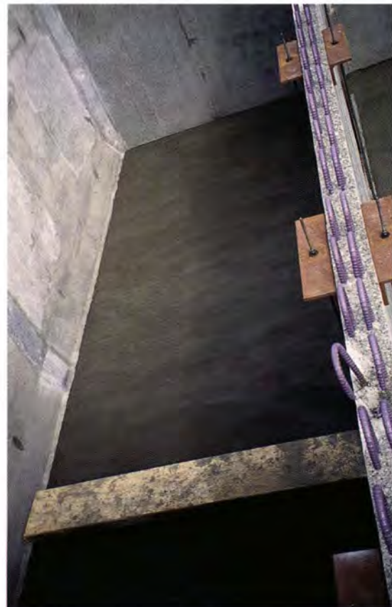
Fig. 18. Cell floor (keel slab) after pouring and finishing.
