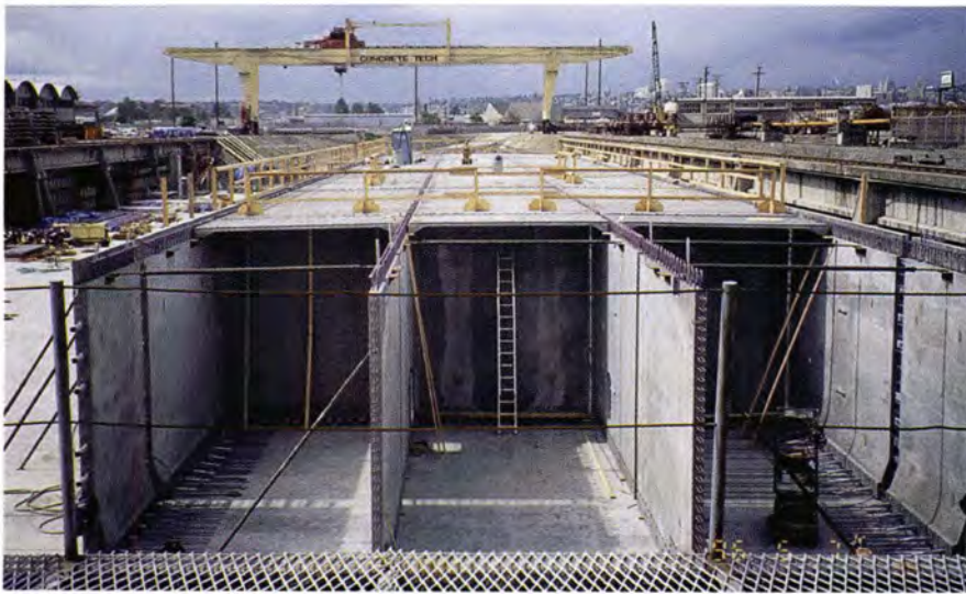
Fig. 16. Assembly of precast components in the graving dock.
