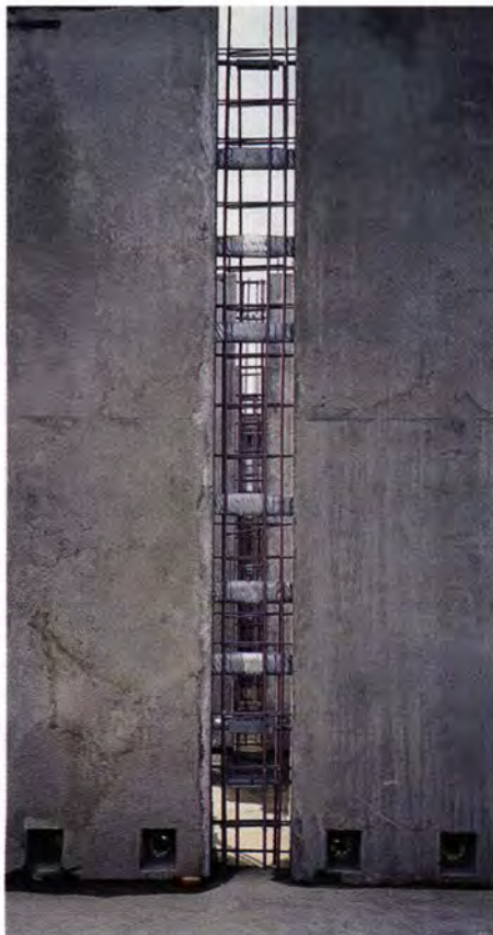
Fig. 17. Interior pilaster with post-tensioning ducts spliced and reinforcing bars tied.
