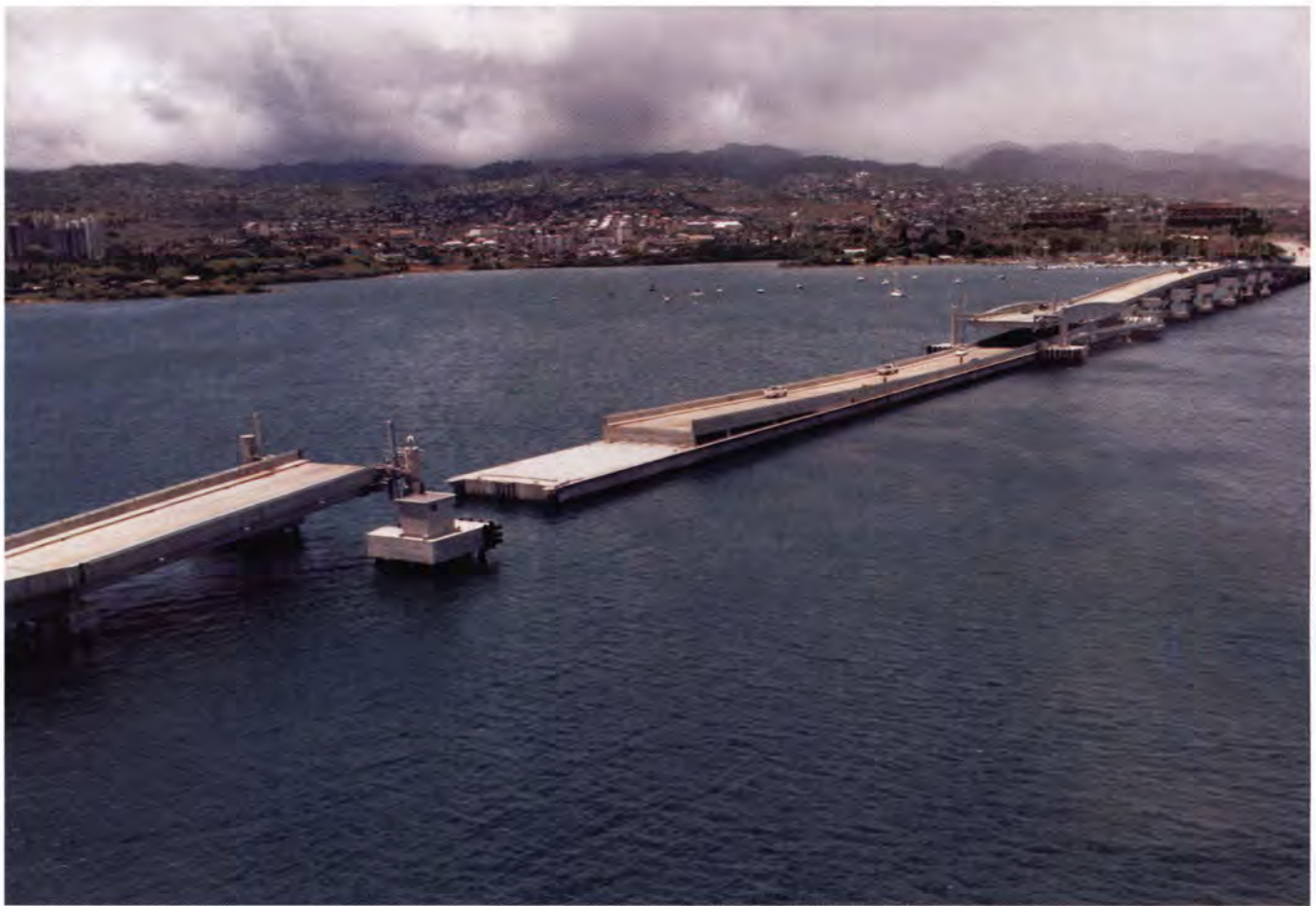
Fig. 2. Precast prestressed floating drawspan showing floating section being retracted under fixed bridge spans. (Courtesy: Williams Photography of Honolulu.)
