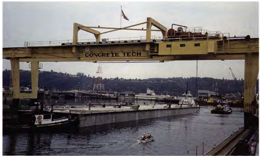
Fig. 26. Maneuvering the pontoon into Puget Sound.
