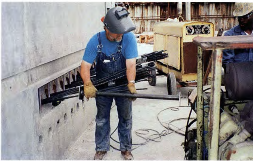
Fig. 22. Pushing post-tensioning strand into the keel ducts.
