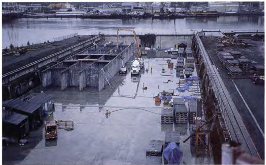
Fig. 19. Pontoon B under construction in the graving dock.
