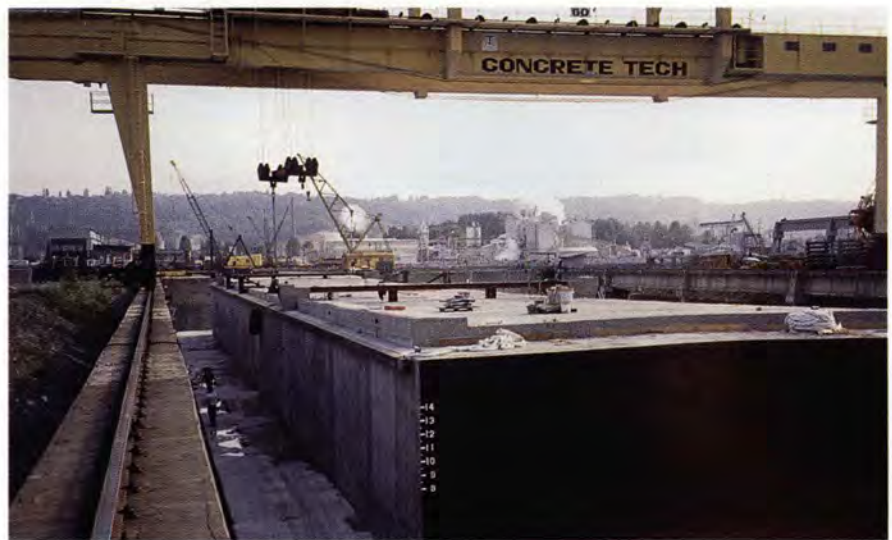
Fig. 25. Pontoon B ready for launching.
