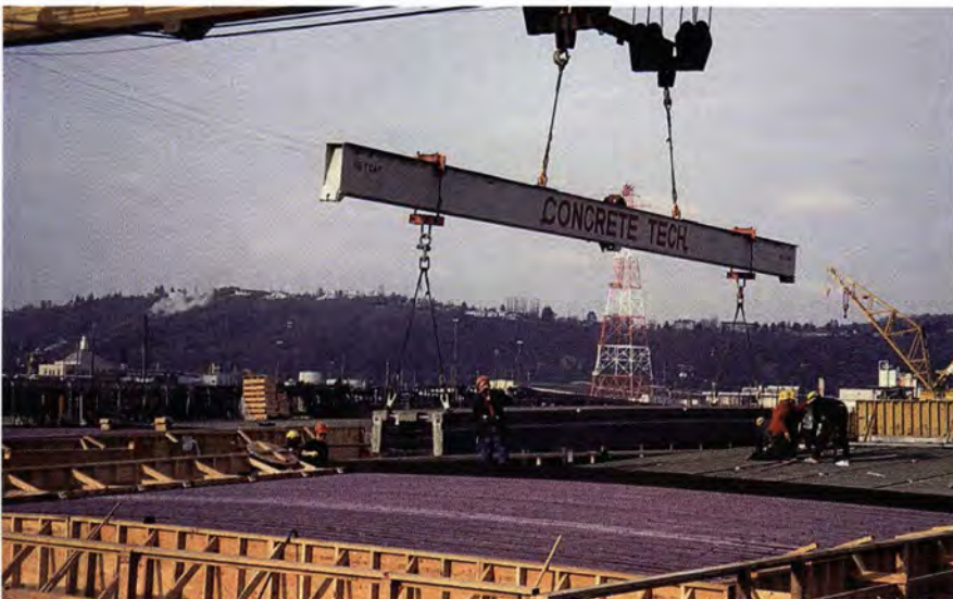
Fig. 23. Erecting channel beams for the elevated superstructure on the pontoon.
