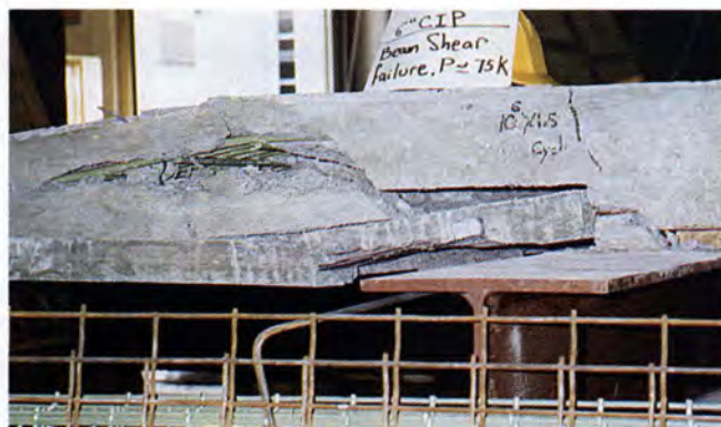
Fig. 17. Shear failure of conventional SIP panel system showing lack of tension tie development due to strand discontinuity.
