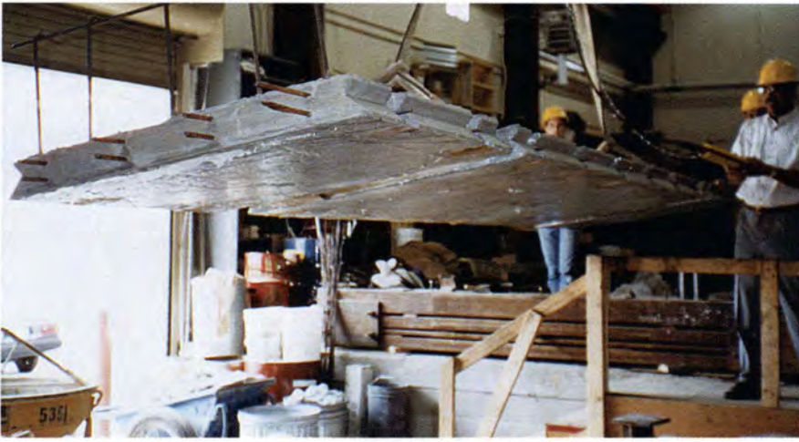
Fig. 11. Precast panel during handling displaying good stiffness.
