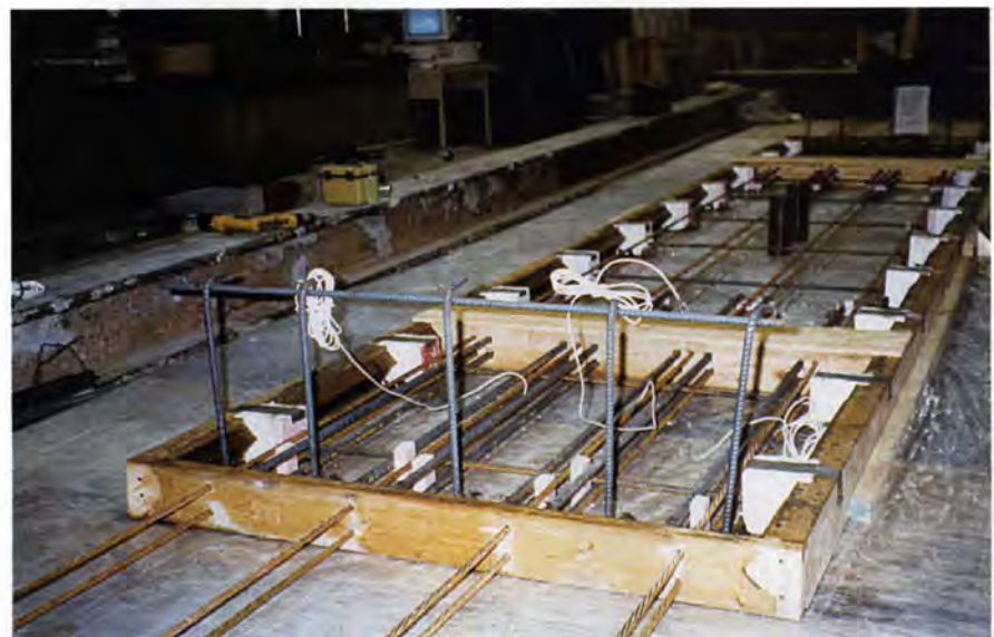
Fig. 10. Details of completed forming.
