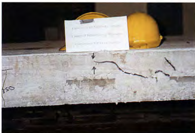
Fig. 16. Flexural cracking at ultimate load.
