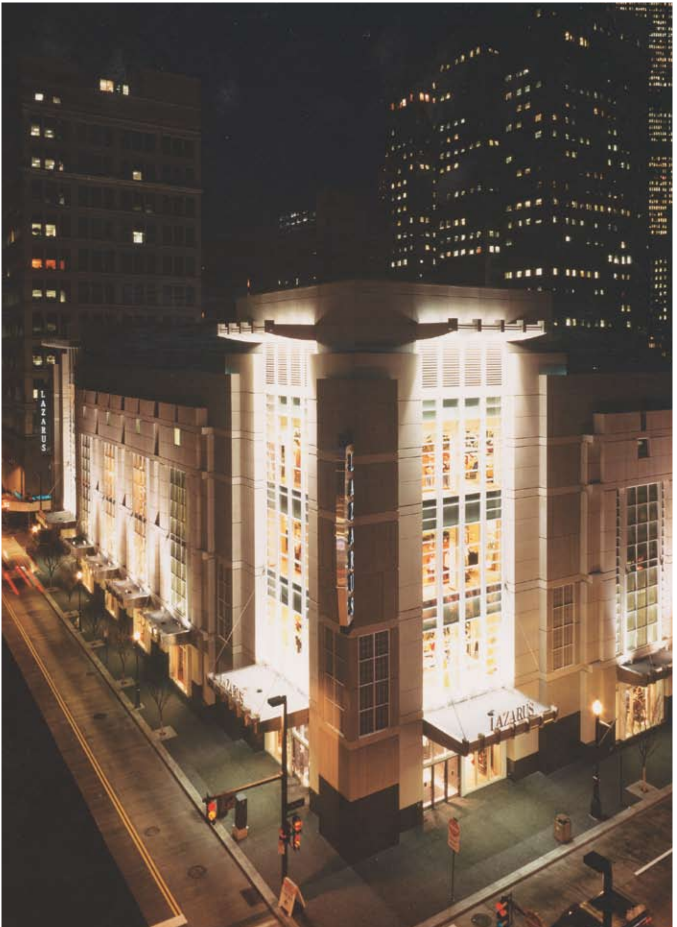
Fig. 13. Bright interior lights highlight the entrance tower of the Lazarus Department Store.
