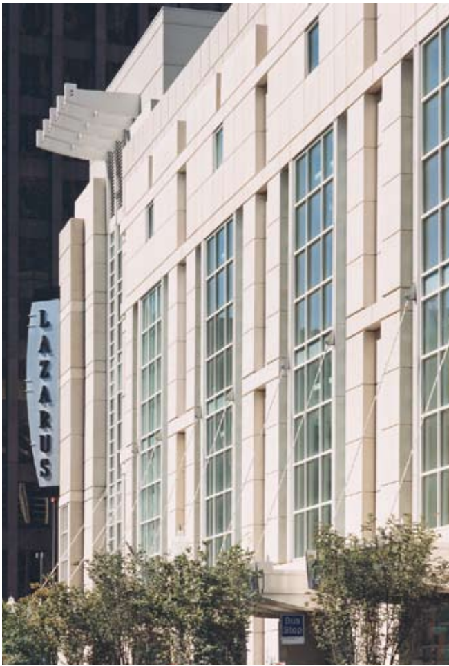
Fig. 8. The outer plane of panels is lighter in tone and serves to frame the tall window bays.
