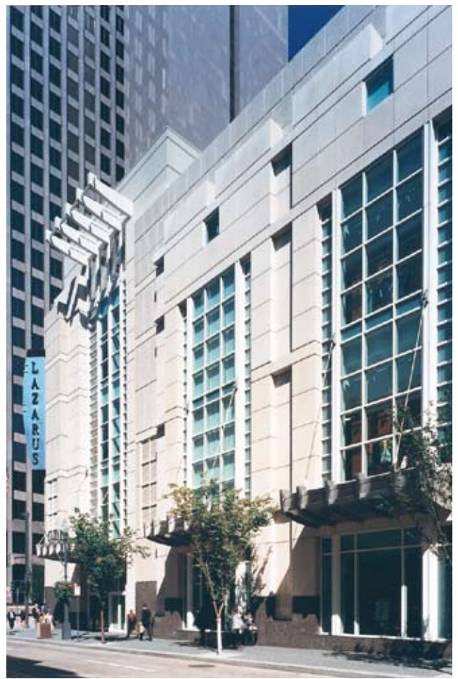
Fig. 9. The second plane of panels features a light sandblast that contrasts with the other layers.
