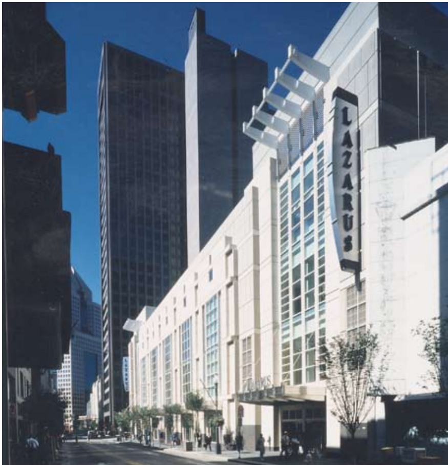
Fig. 5. Rustication and textures on the precast panels help the luxury store fit in with its neighboring buildings, built in the 1900s.
