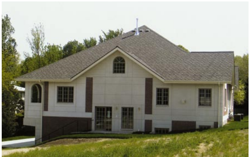
This duplex in Omaha, Neb., features precast concrete wall panels, flooring and roof beams, producing a sturdier home that's pleasing to the eye.
