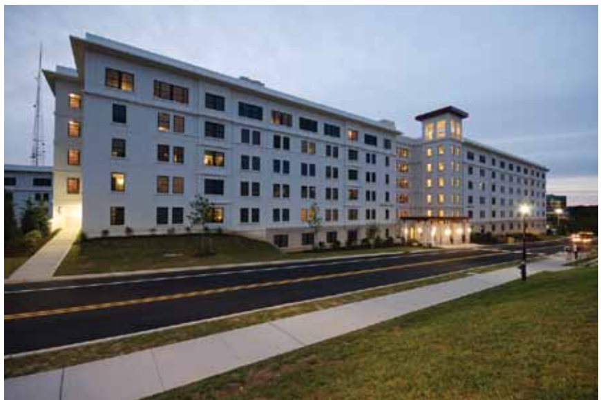
The total-precast concrete structural solution consisted of load-bearing precast concrete wall panels and hollow-core floor planks. The wall panels feature 3 inches of rigid-foam insulation secured with proprietary carbon-fiber shear trusses to minimize thermal bridging while transferring shear forces between the layers.
