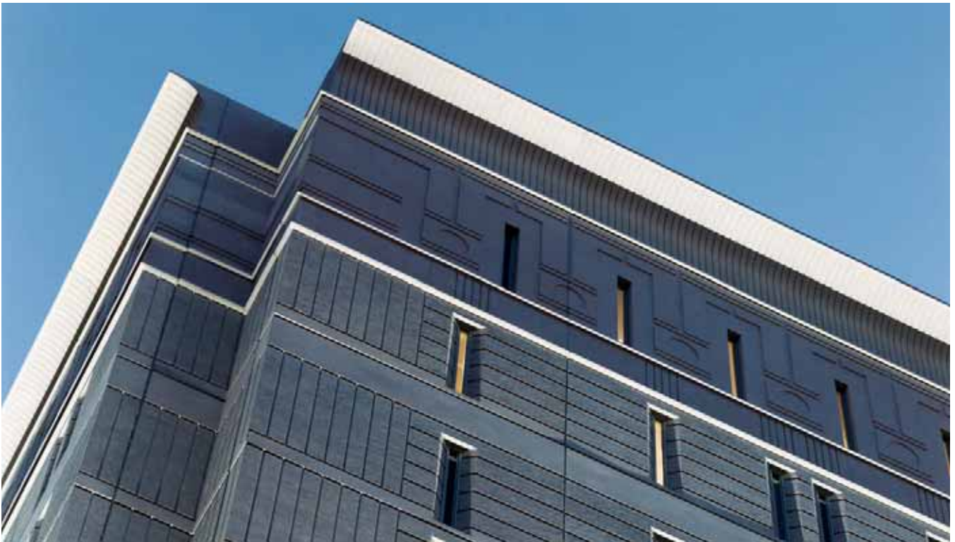
Fig. 21. The elegantly detailed cornice features a 3 ft (0.914 m) radius that adds interest and hides mechanical equipment on the roof. Photo courtesy: Jeffrey Totaro.
