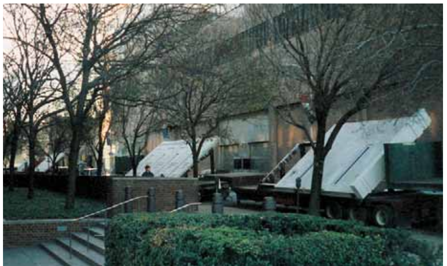
Fig. 17. Because of a lack of staging area, trucks sometimes backed up along a parking lane in front of the correction center. Photo courtesy: Jeffrey Totaro.
