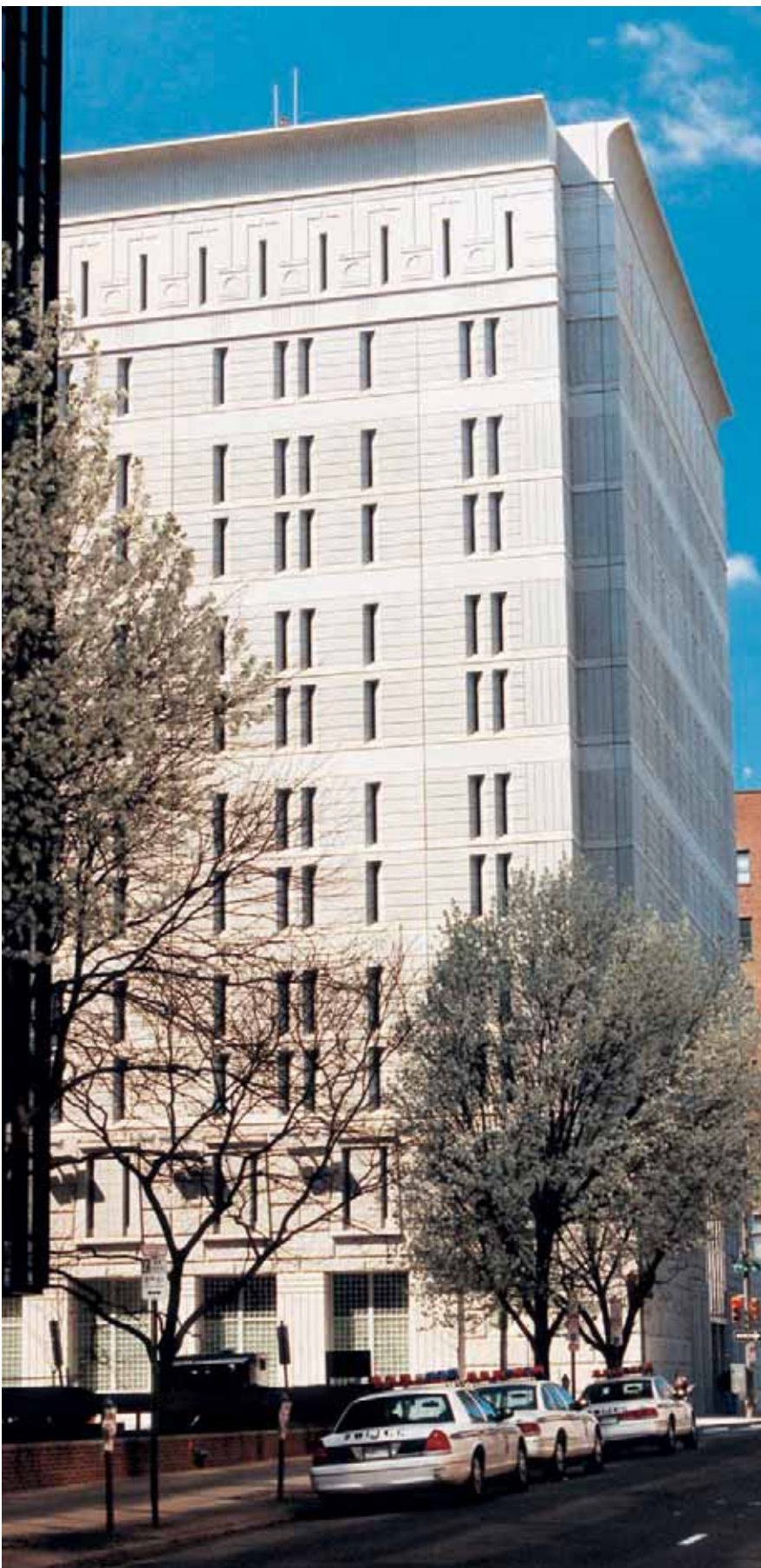
Fig. 1. The new Federal Metropolitan Detention Center in downtown Philadelphia with its cladding of architectural precast concrete panels. Photo courtesy: Robert Meier.
