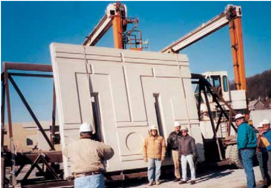
Fig. 11. Finished window panel at precaster's yard.
