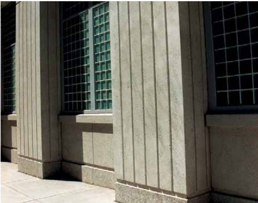
Fig. 6. A column along the building's base shows the variety of detail achieved on a low budget. Photo courtesy: Robert Meier.
