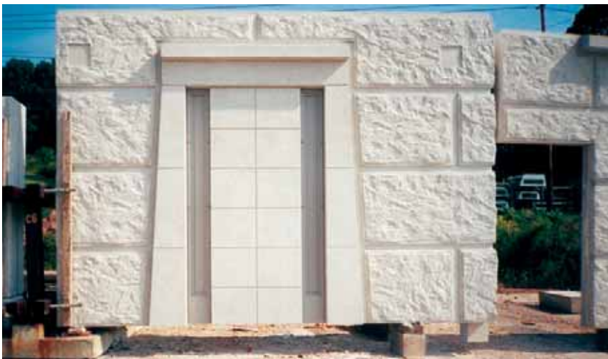
Fig. 12. Finished wall panel for lower levels at precaster's yard.
