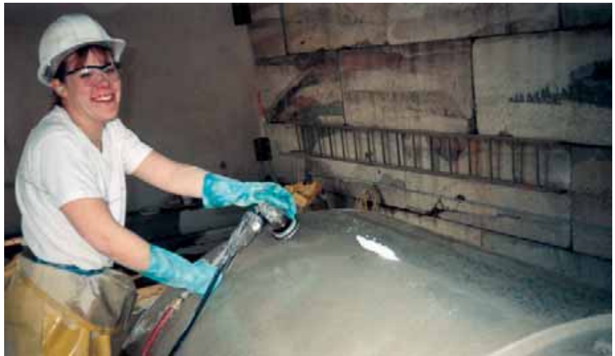
Fig. 8. Several precast concrete columns had to be hand polished – a highly skillful procedure which made the columns look very elegant. Photo courtesy: Jeffrey Totaro.
