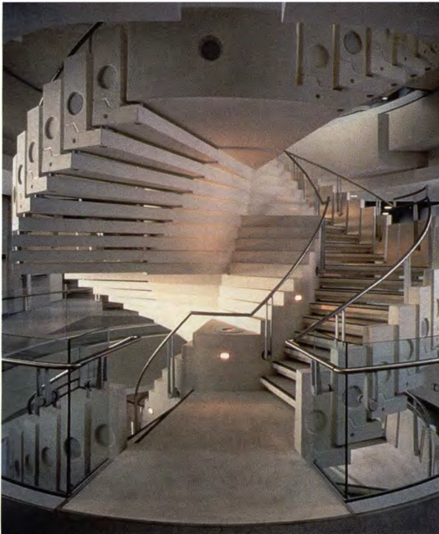
Fig. 17. Landing components provided at each level are the only deviation from the typical dimensions cast for the propeller-shaped precast units.
