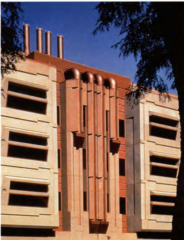
Fig. 4. The laboratories' exhaust ducts were left exposed on the exterior, creating an additional design element and serving as a vertical break between façade sections.
