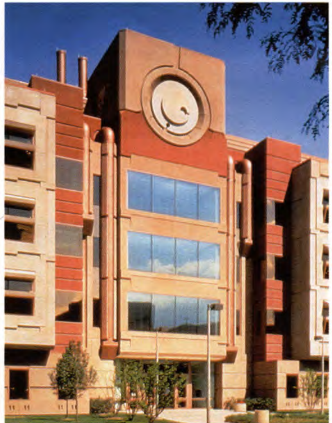
Fig. 5. Distinctive precast concrete details were included both inside and out, including the "atomic clock" in the entry tower.
