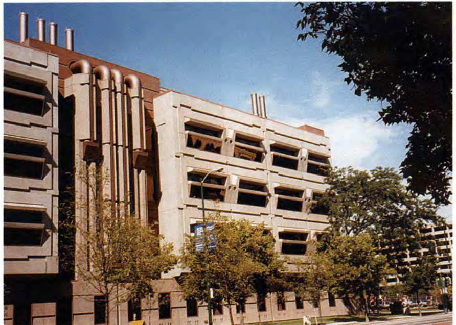
Fig. 8. The two-piece façade panels join with amber-tinted window glass to create striking designs for the fenestration in addition to offering energy-efficient shielding.
