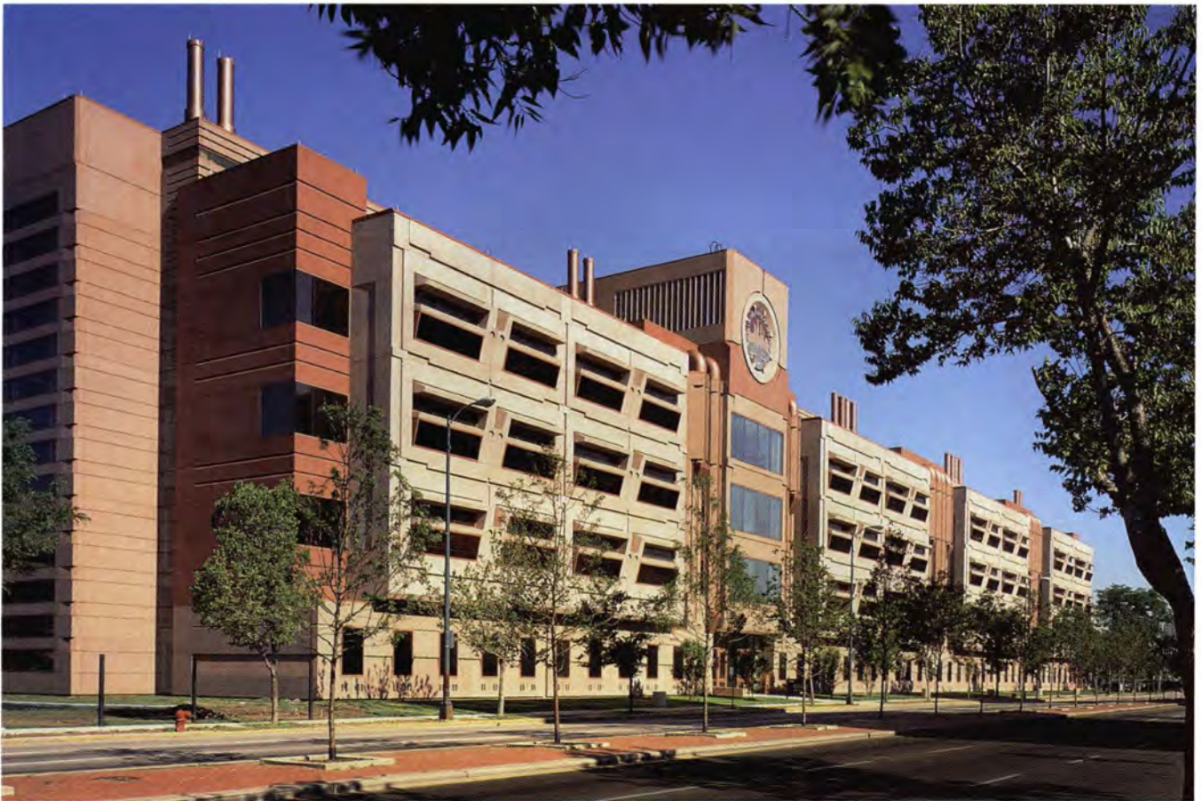
Fig.1. The new Molecular Biology Research Building on the downtown Chicago campus of the University of Illinois took advantage of precast concrete's plasticity to express different building functions on the façade.
