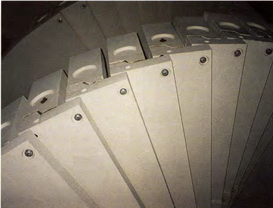
Fig. 18. The casting process for the stair treads was complicated by the fact that all six sides were visible from some angle in the structure.
