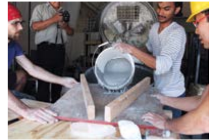
Students working on semi-rigid form work to allow more 3D shapes and new design applications.
