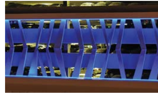
COLORFUL DISPLAY The building's metal panels can be illuminated with programmable LED fixtures that can change the lighting's intensity and color as desired. Photo: Robert Giordano/Design216.
