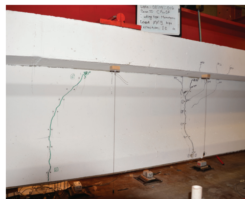
Initial crack pattern
